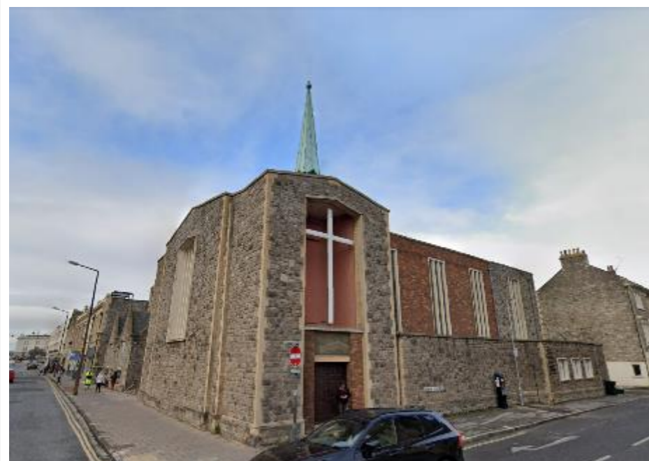
Former Burtons, 31-35 High Street
